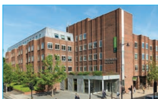
No.5 | Premier House, Twickenham
