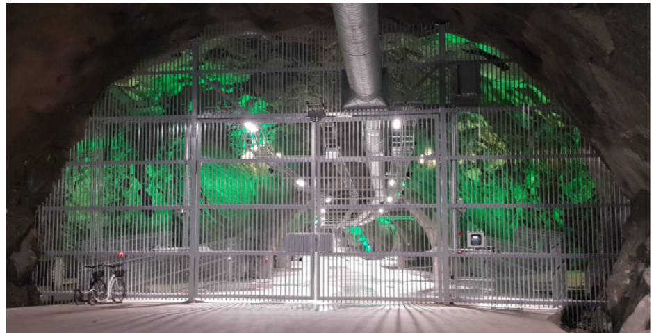
The Lefdal Mine Datacenter in Norway. Source: Lefdal
